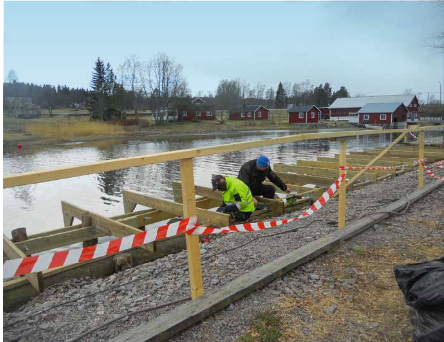
▲ Building a new pontoon in Tynderö.
